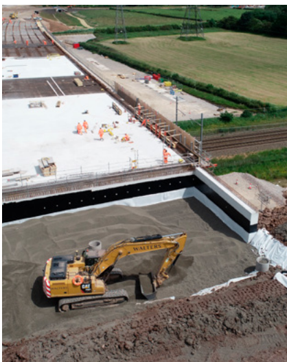
LECA LWA's robust lightweight properties provided the key solution for poor ground-work conditions
