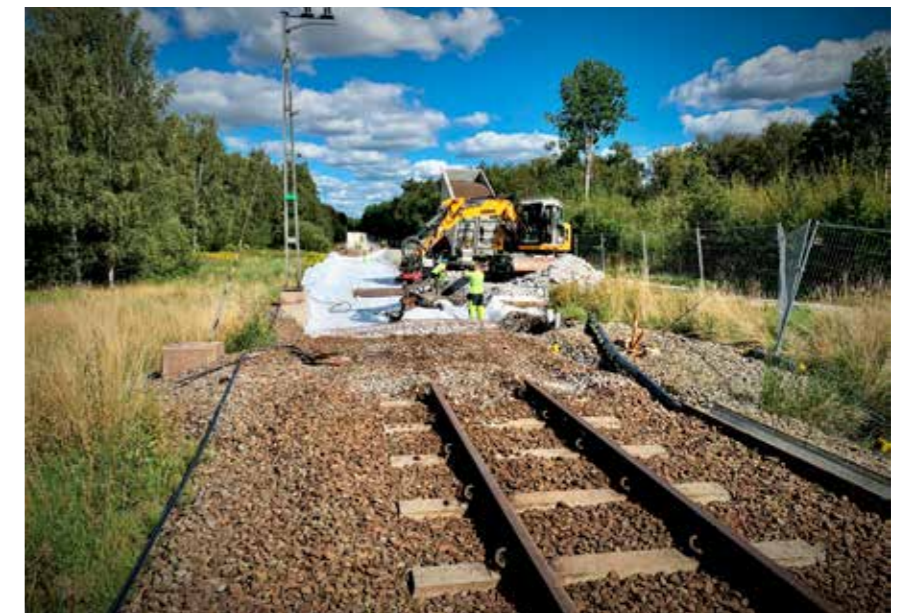
Geotextile was placed at the bottom of the solution.
