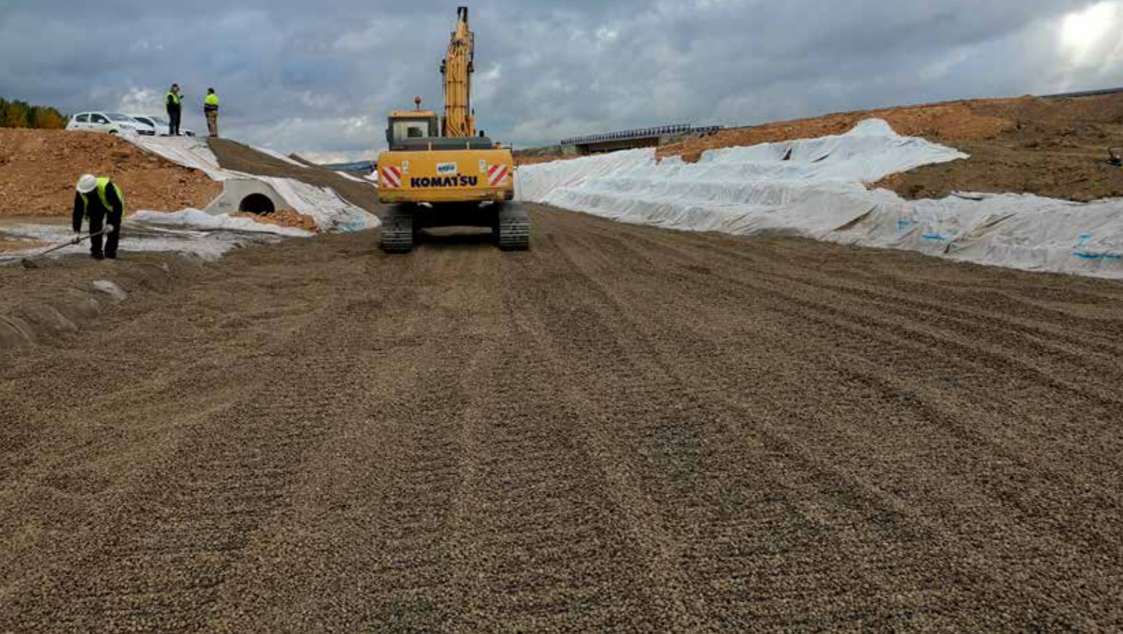
Spreading and compaction process.
