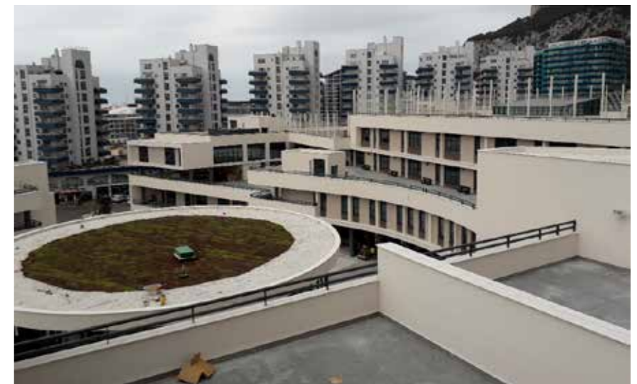
A total of 430 thousand assorted Isoargila® blocks were used to construct the two buildings.
