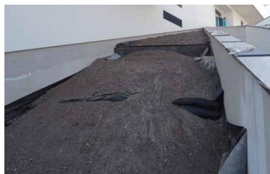
Scarps made of expanded clay "mattresses"
