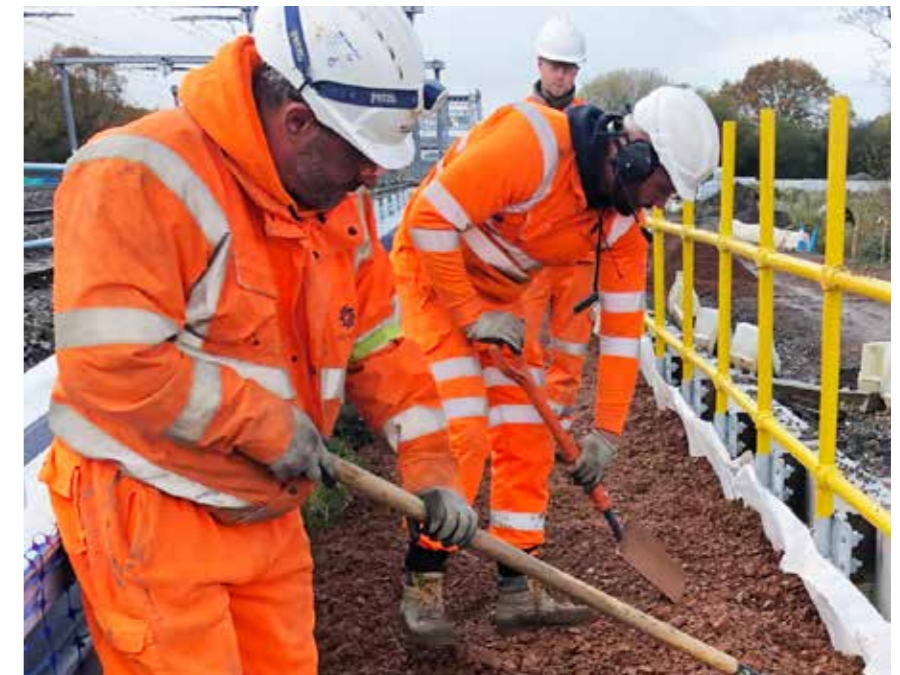
The Leca LWA (10-20mm) was delivered loose by Walking Floor trailers
