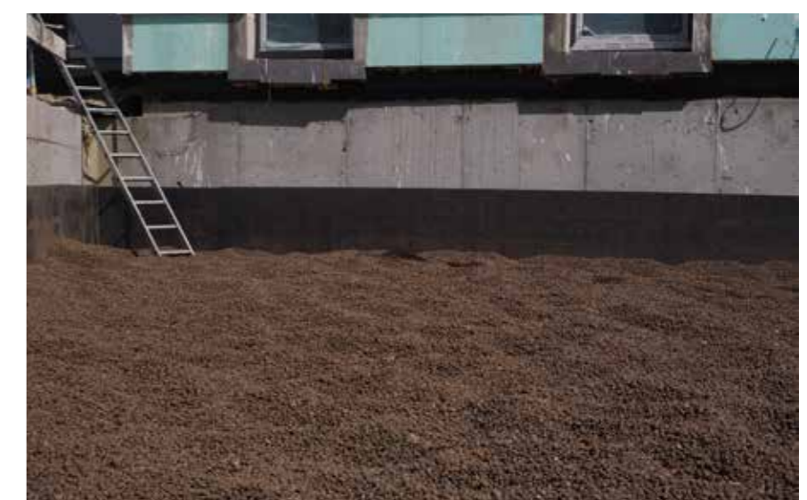
Filling adjacent to the building and retaining walls
