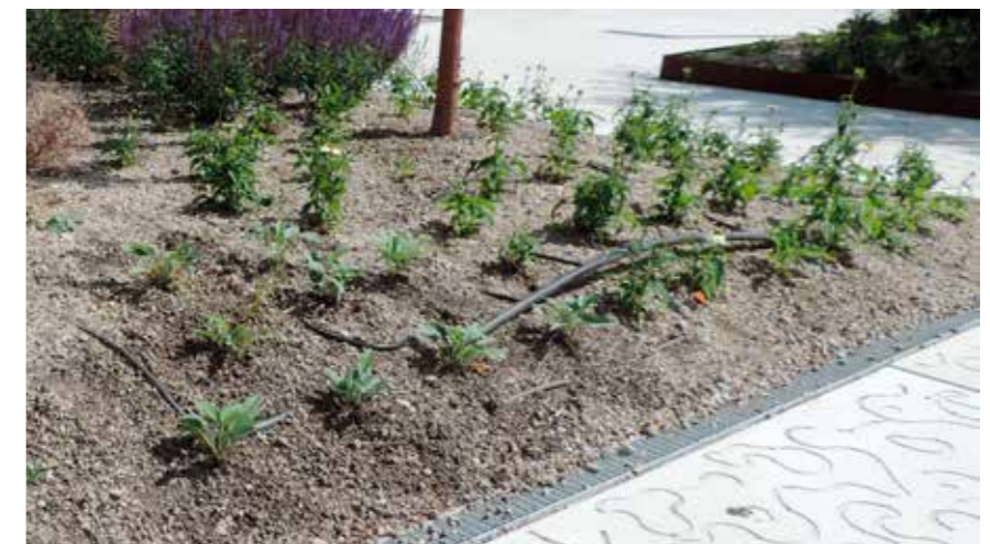
The irrigation system exists of 6 km of water hose, laying in the soil in the green areas.
