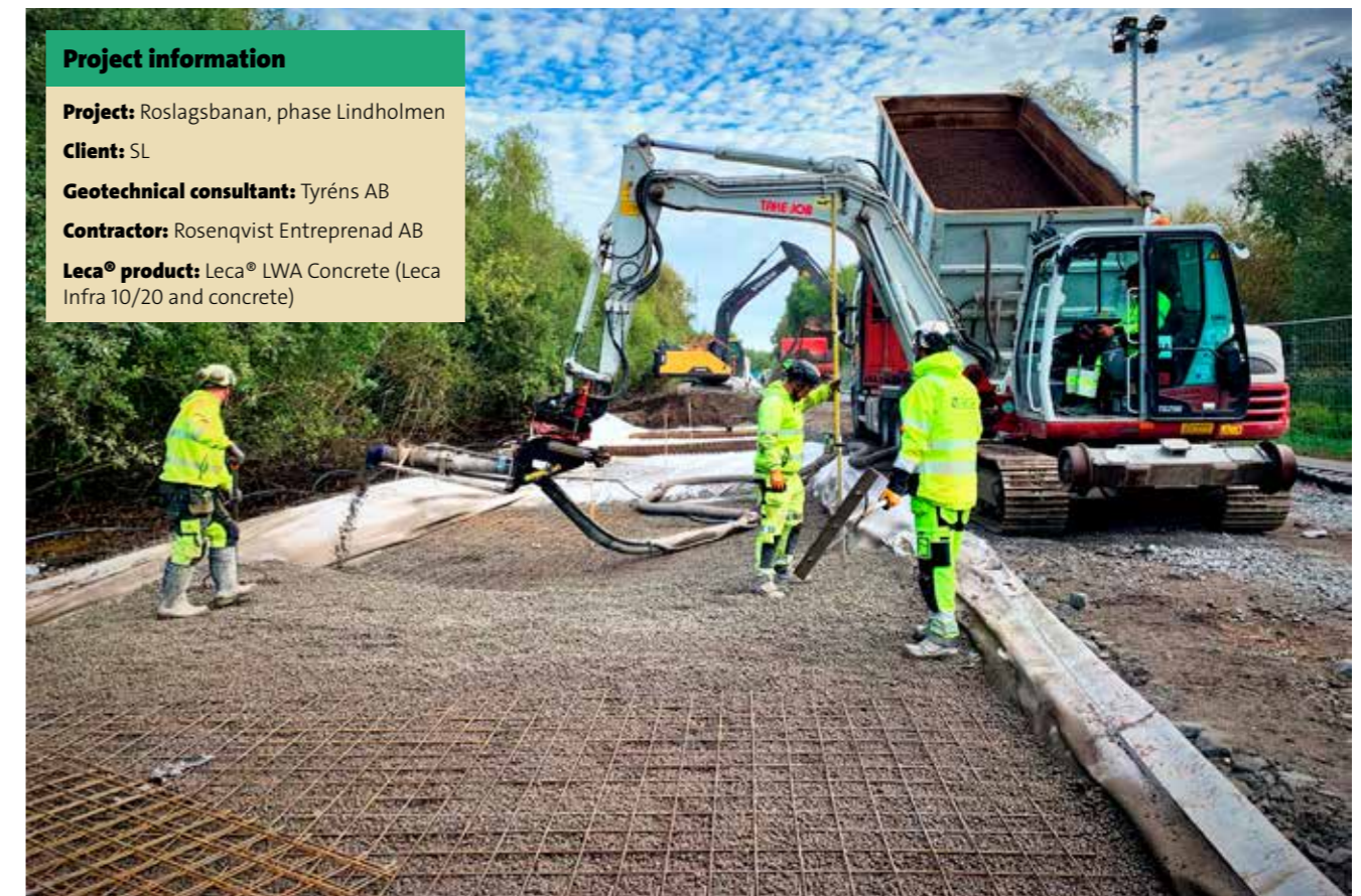
LLP is an innovative solution achieved by combining Leca LWA and cement mixture by using a specially developed nozzle.
