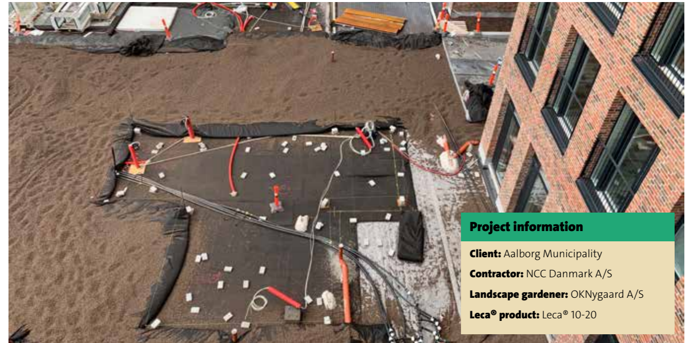
When the Leca LWA was laid out the geotextile was folded over it, so the material was locked on the sloping areas.
