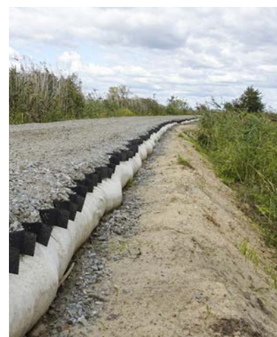
Next, a 20 cm thick surface layer made of 0–31.5 mm aggregate was laid within a geogrid.
