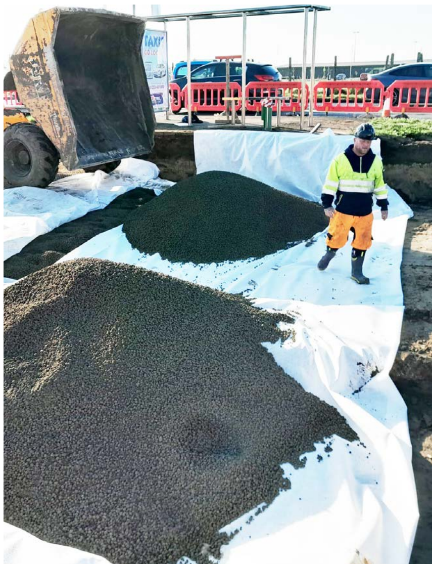
Leca LWA was chosen as a lightweight fill material, significantly reducing load-induced settlement.
