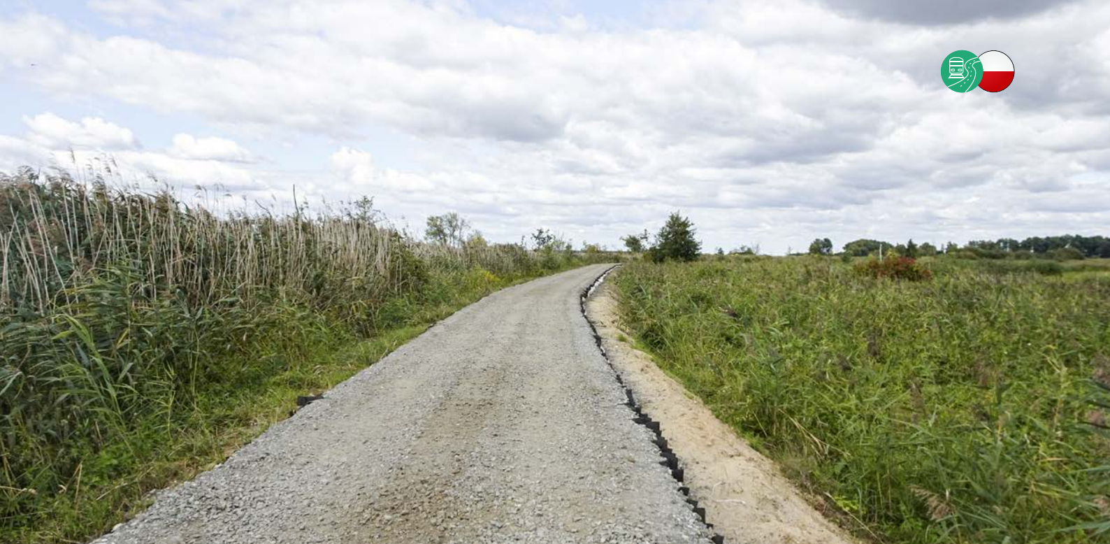
Leca LWA Geotechnical 8/10-20 RX is several times lighter than natural aggregates or soil.
