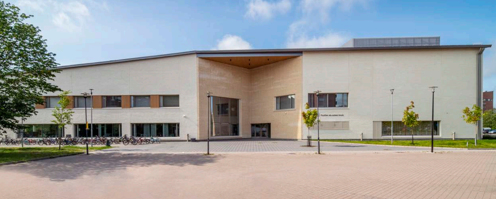
The newly built Puotila school provides a sustainable and spacious setting for students.
