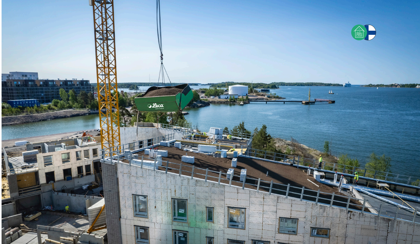
Lightweight aggregate was delivered to the roof (5–9 storeys) using a lifting box, supporting efficient installation on site.
