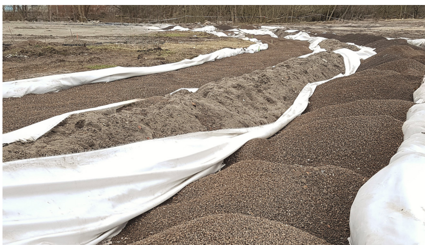
Compacted Leca LWA (8/10mm–20mm) in geosynthetic material forms load-reducing “expanded clay aggregate mattresses”.
