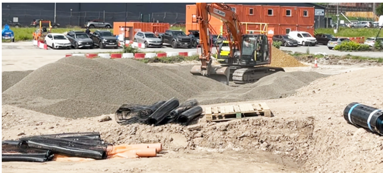
3,000 m 3 of Leca LWA used in retaining walls for a new elevated pedestrian walkway.
