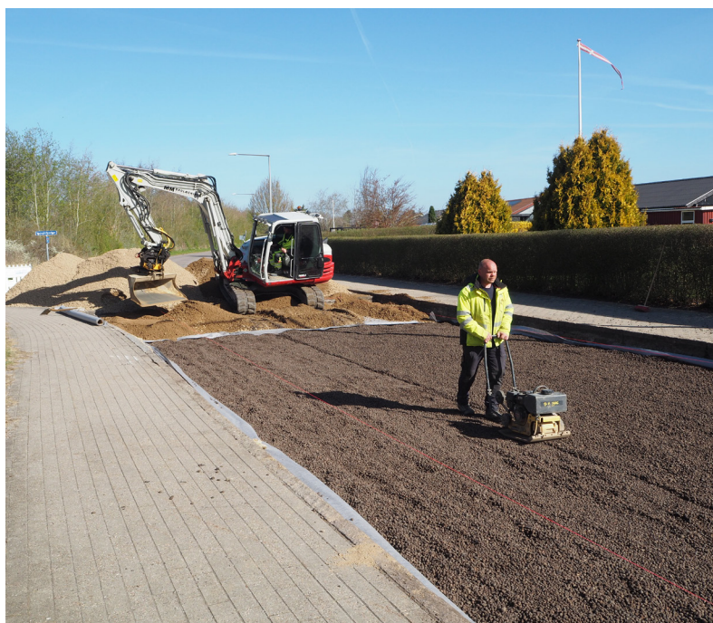
Leca LWA replaces sand as bottom protection
