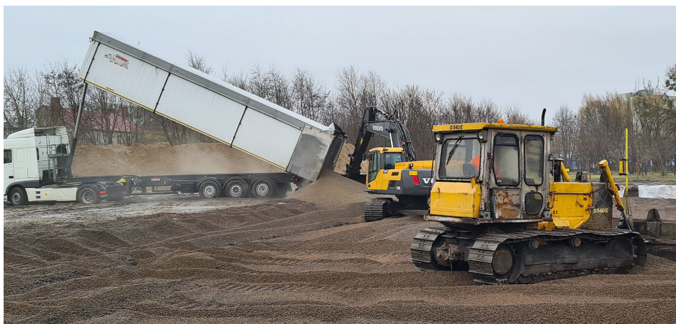
The Leca LWA was delivered by tipping truck, enabling fast and efficient installation directly on site.
