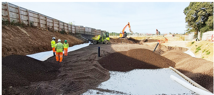
Over 5,600m 3 of Leca LWA supported the culvert extension before earthworks began.
