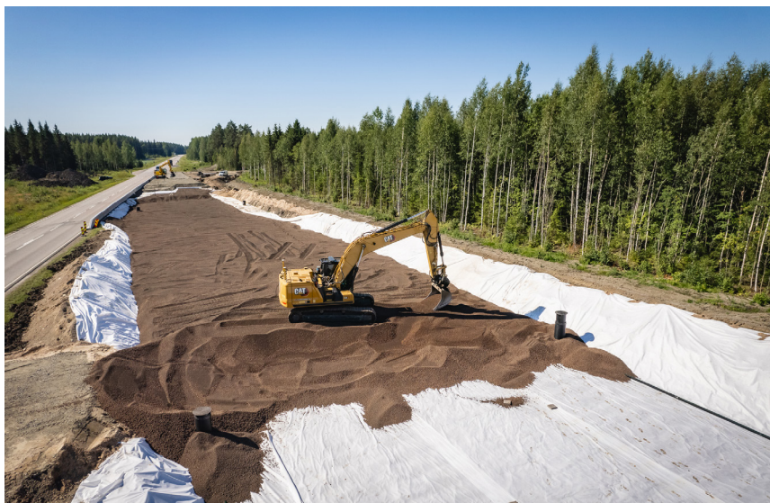
Leca LWA layer 1.3–3.3 m, enclosed in geotextile.
