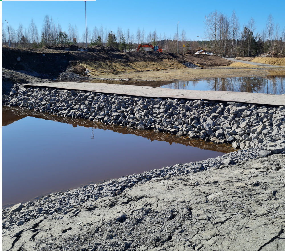
Completed dam filters water before discharge.
