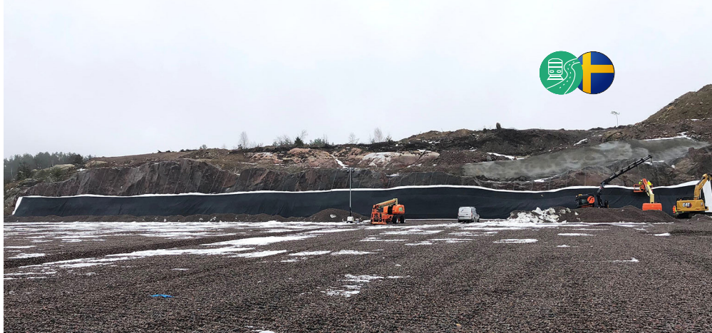
Completed section of the containment structure along the former quarry, ready for the next stage.
