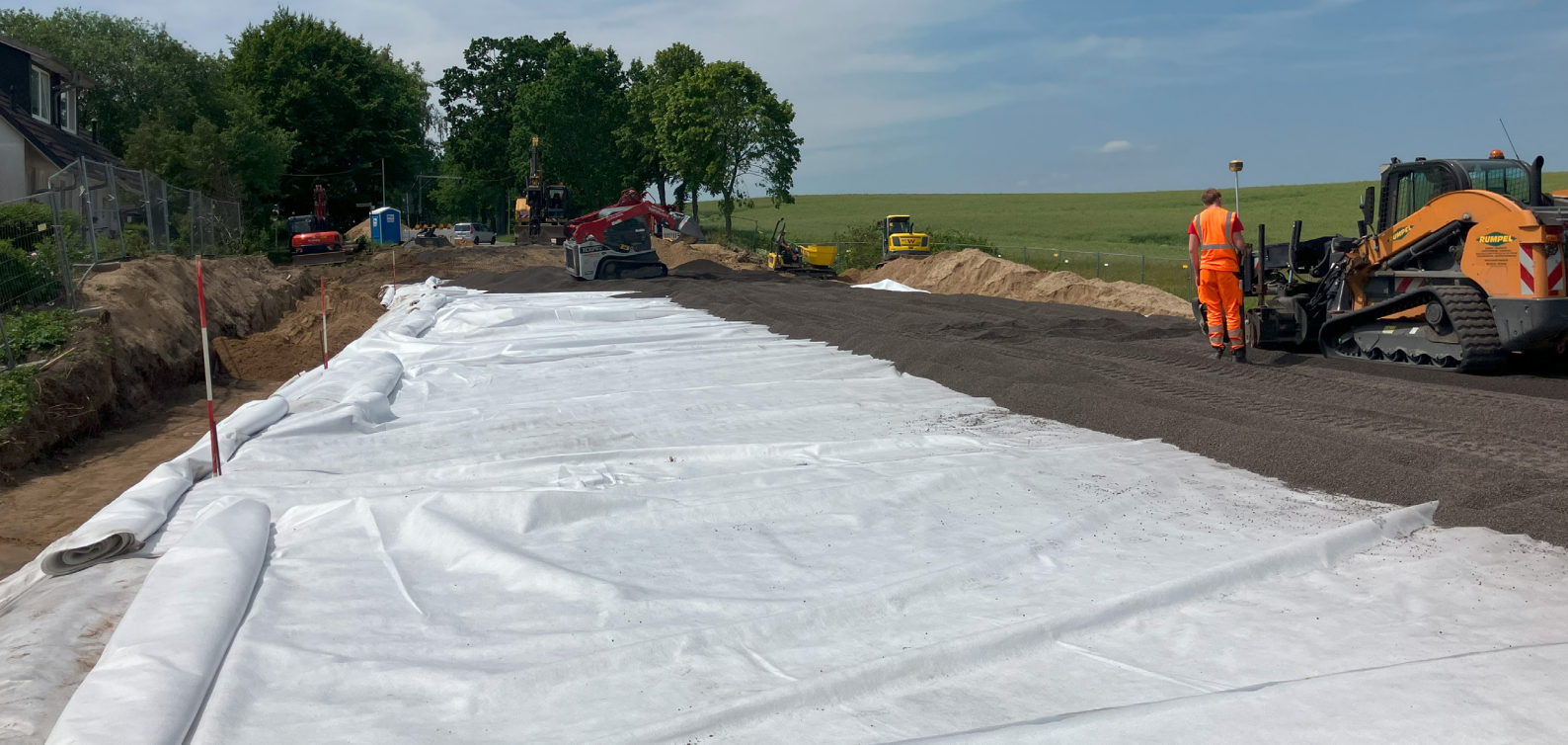
Leca LWA was enclosed in a geotextile
