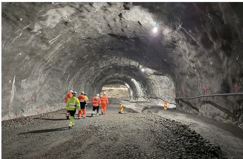
Project team on site in the Brattfjelltunnel, where LWA is used for frost protection and drainage
