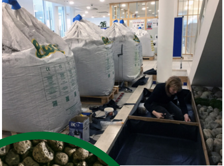
Arja Rantasalo makes sure that the tanks are water proofed before adding Leca aggregate and water.
