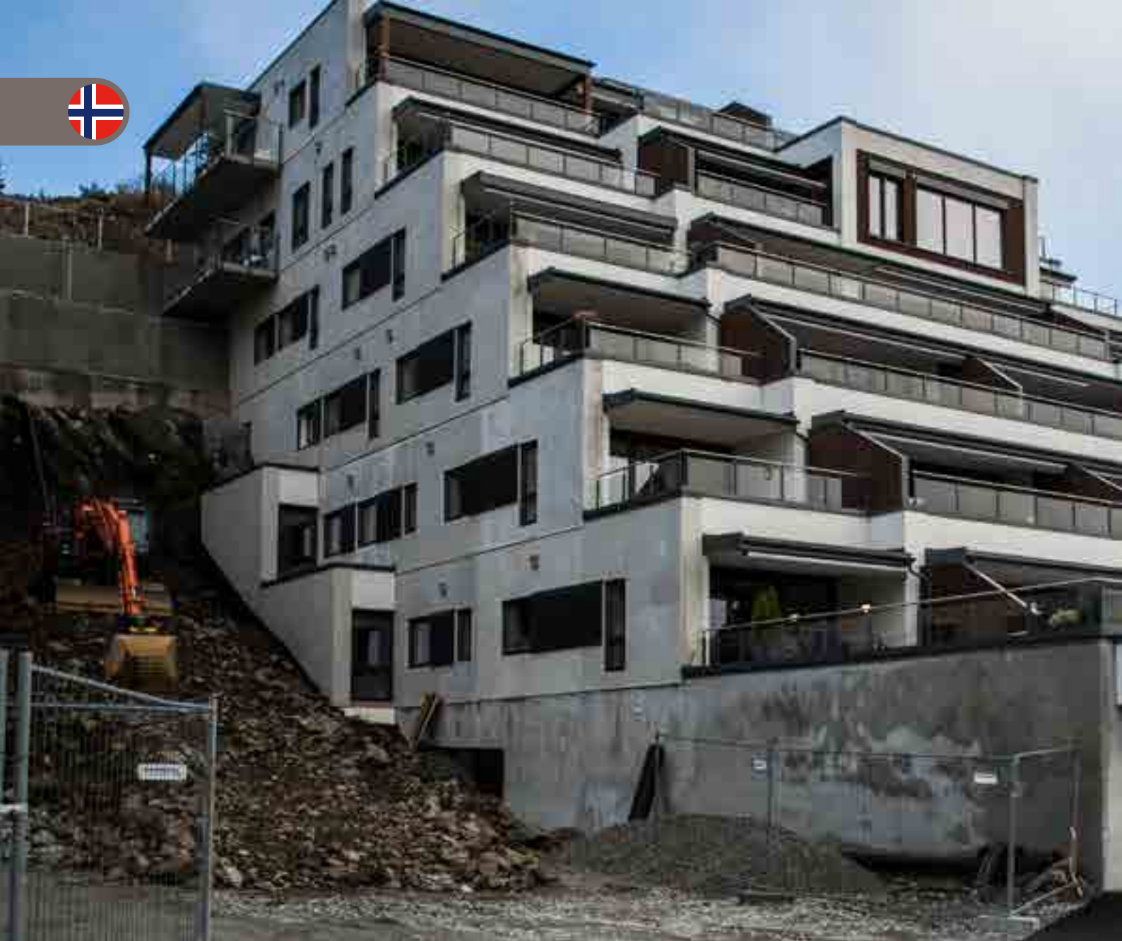
One of three blocks being built in Hokksund by Betonmast Telemark.
