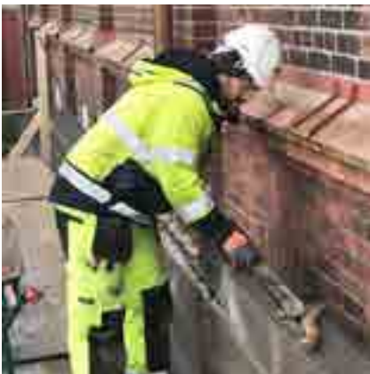
The builders have had a positive experience of constructing the firewall.
