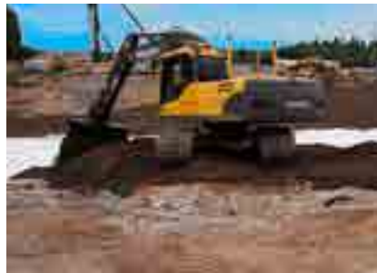
The lightweight structure was compressed in approximately 0.5 m layers.
