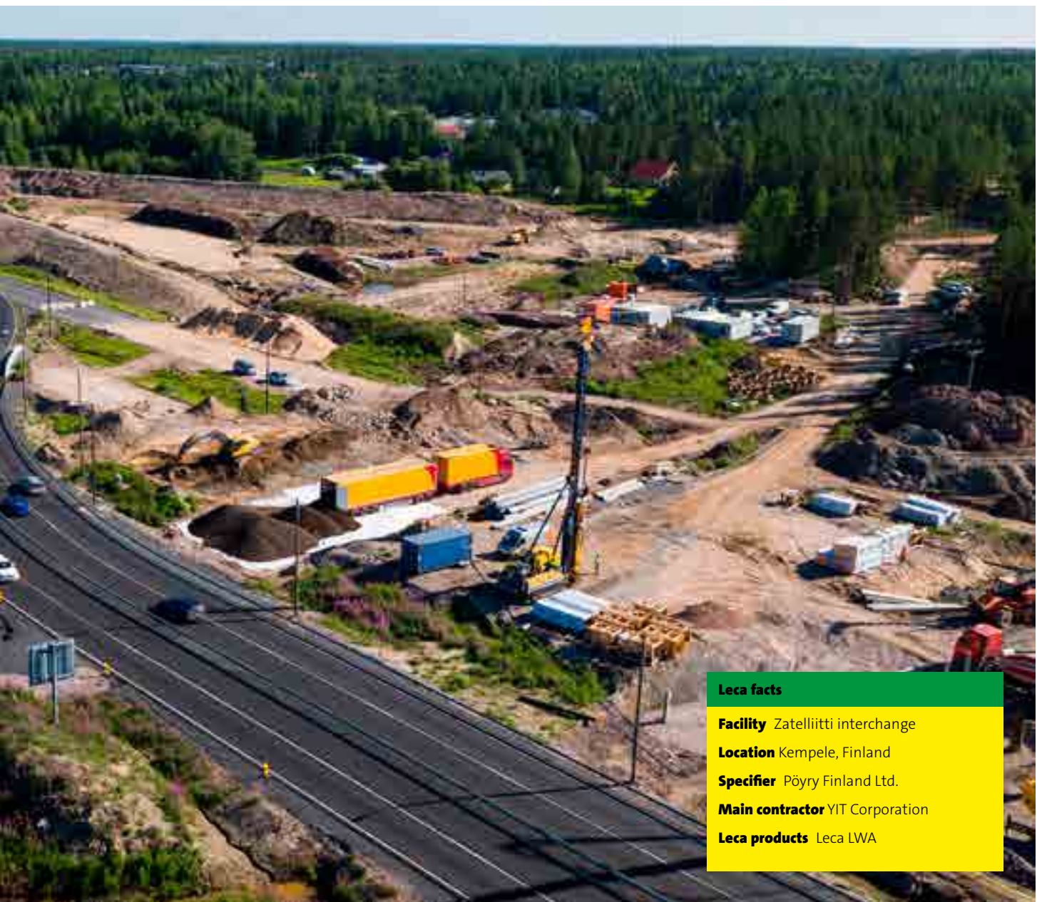
The lightweight structure was compressed in approximately 0.5 m layers.
