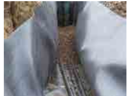
Electric cables laid in the geotextile filled with loose Leca LWA.
