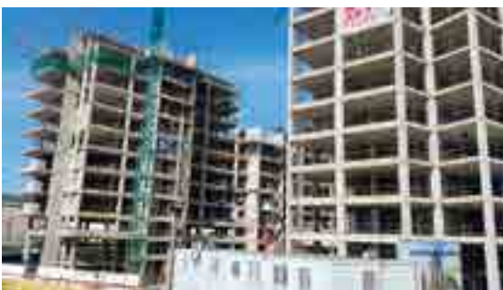
Building before the placement of Leca blocks.
