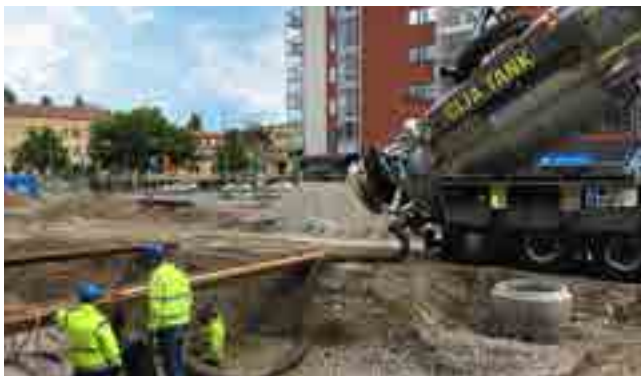
The material was quickly blown in using a pneumatic blowing vehicle.
