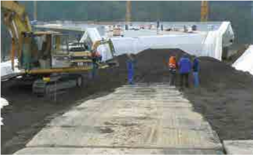
Road and bridge joints built with Leca LWA
