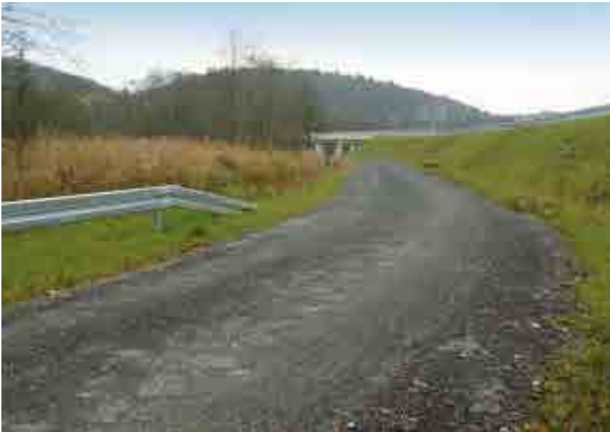
It was necessary to build several service roads.
