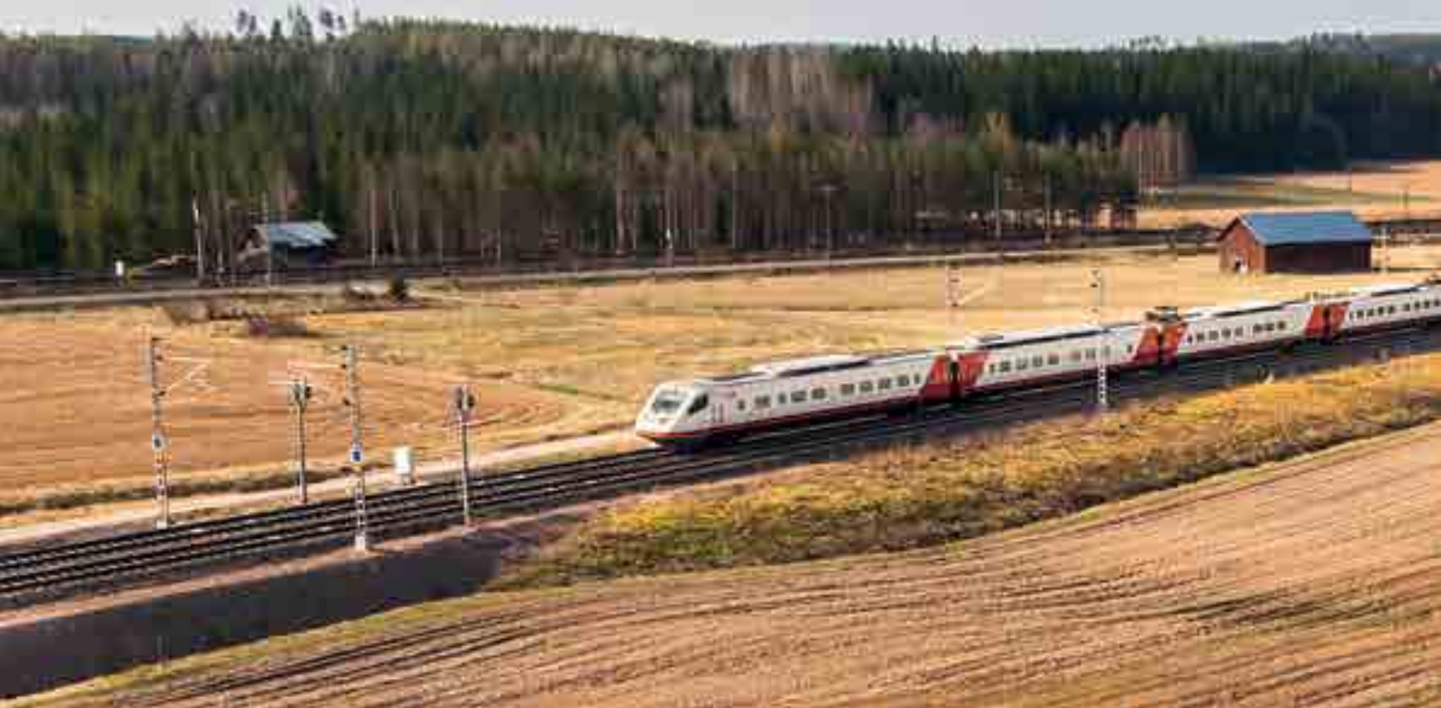
A high-speed railway between Kerava and Lahti is partly constructed in low-lying areas with thick soft soil layers
