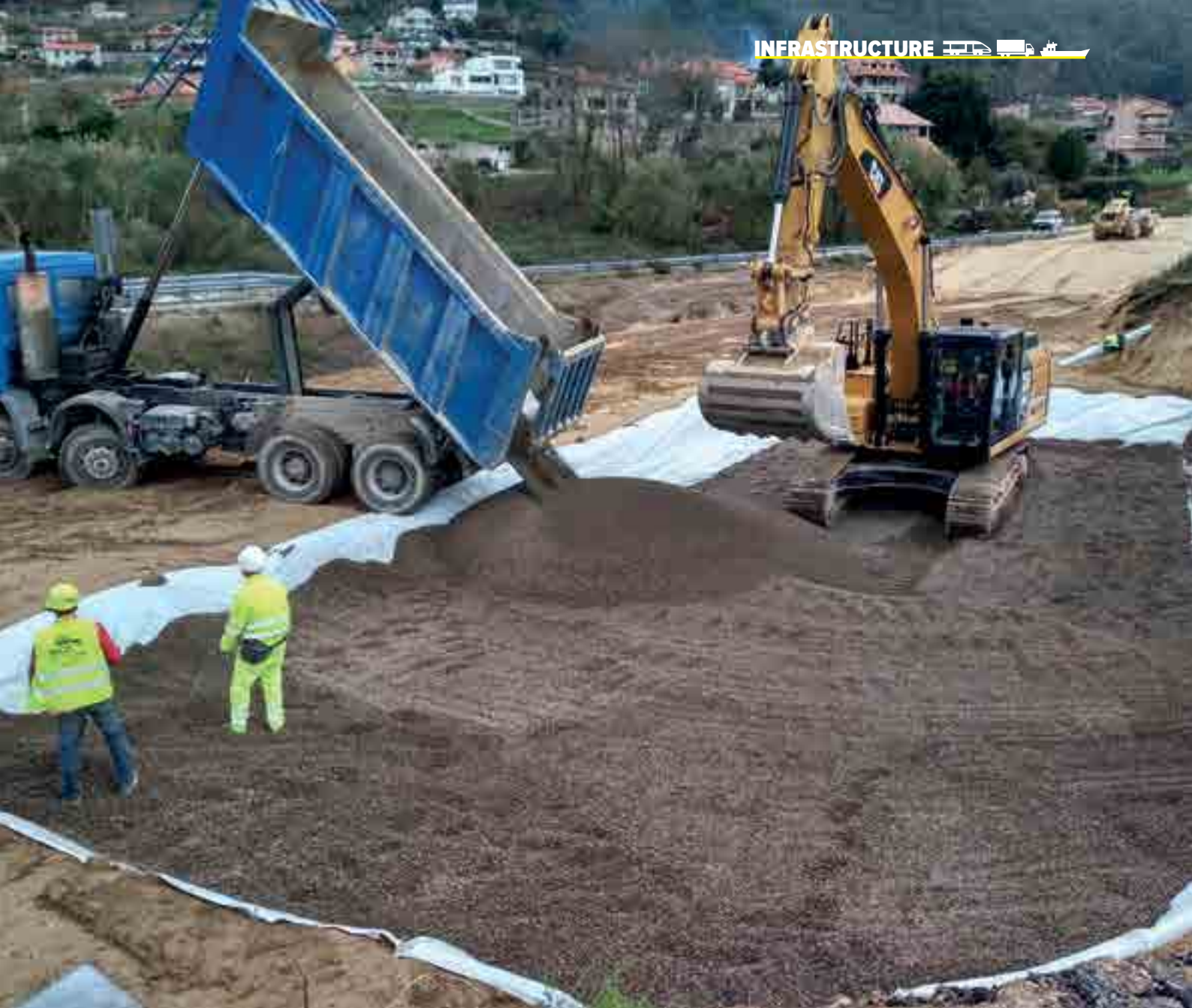
Installation of Arlita® on the structure.
