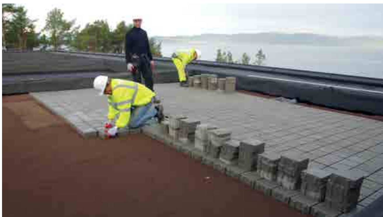
The crushed Leca-material is hidden below the pavers in the blue-grey water management pilot at Høvringen in Norway.
