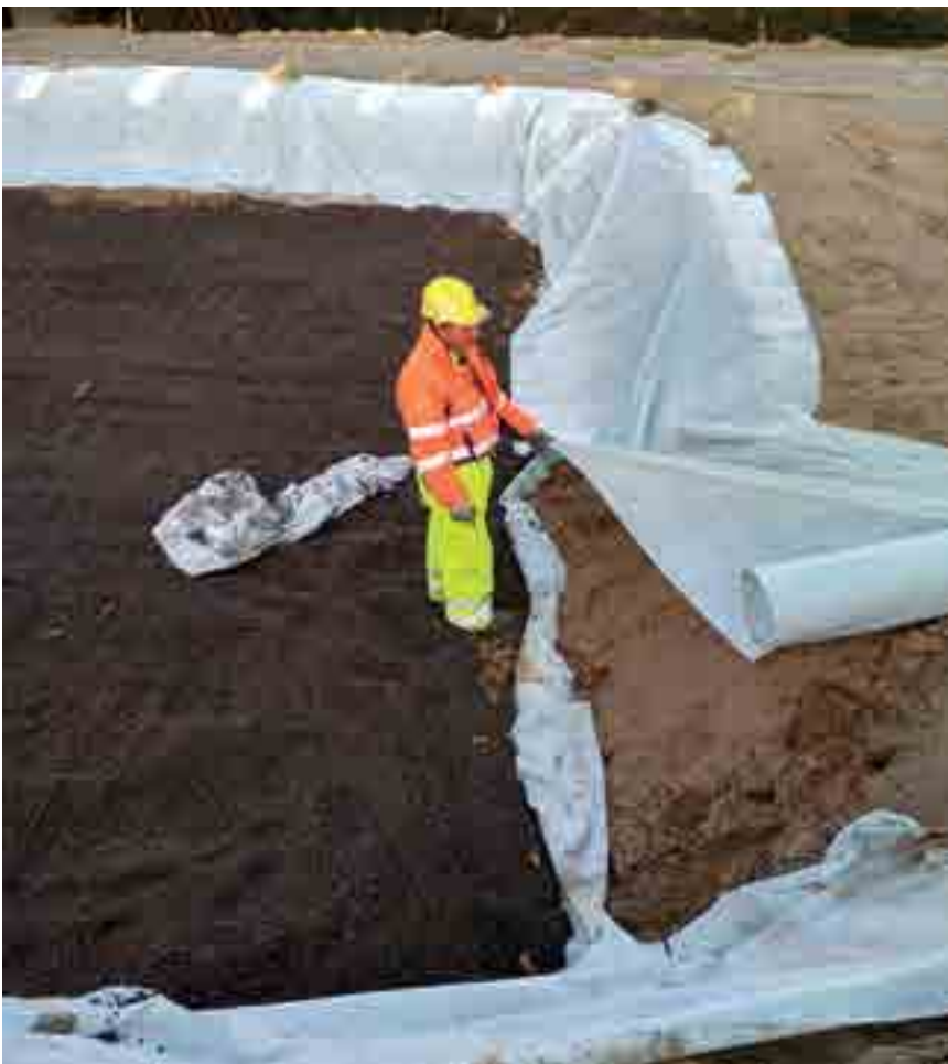
Polypropylene Geotextile installation (250 gr/m 2 ).
