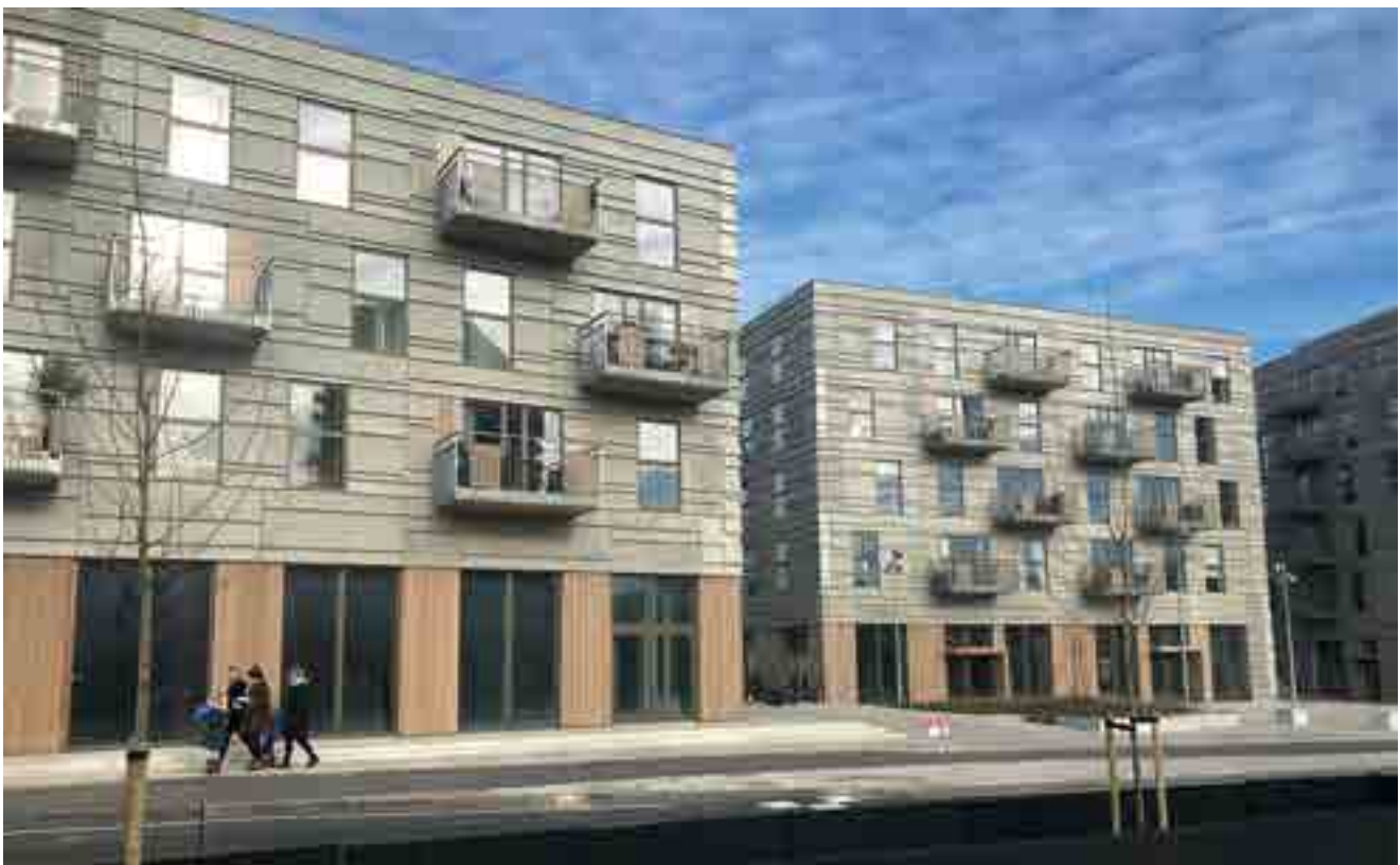
LWA was used for drainage in the basement and on top of a parking garage.
