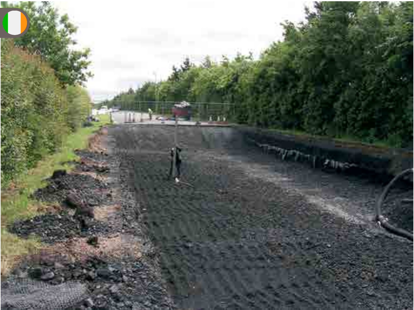
Leca LWA was used to replace heavy road construction material.
