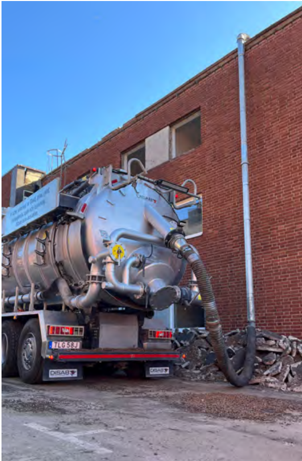
The truck was easily set up right next to the building.
