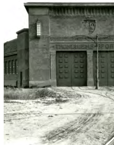
The old tram stables at Dalsenget in Trondheim were built in 1923. In 1956, large parts of the building burned down along with most of the rolling stock of what was then Trondheim Sporvei (Photo: Trondheim city archive, photographer unknown)
