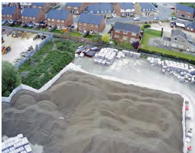
The project minimized environmental impact by sourcing LECA LWA from a location less than 10 miles away
