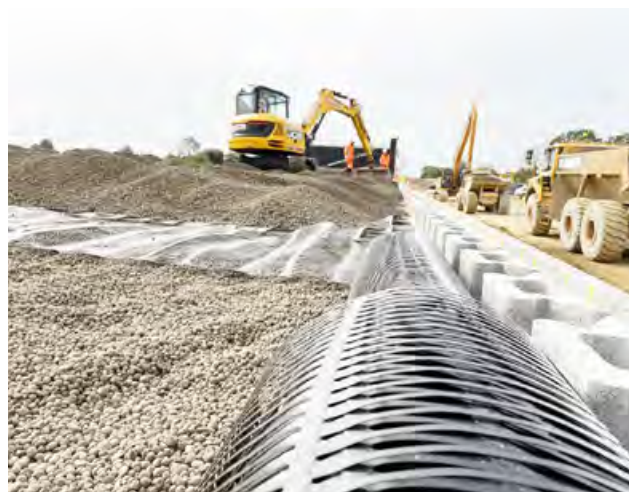
Innovation Meets Infrastructure: The Synergy of LECA LWA and the Tensar Grid System in Spalding
