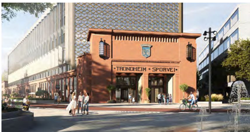
In addition to being Trondheim’s largest office workplace, “Teknostallen” will also contain a fitness center, shops, restaurants and a 3,000 m 2 glassed-in year-round garden, eateries and a 3000 m 2 glassed-in year-round garden (Illustration: KLP Eiendom)
