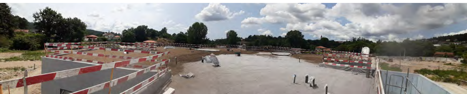
Approximately 250 m 3 were applied to the building's roof through direct pumping.
