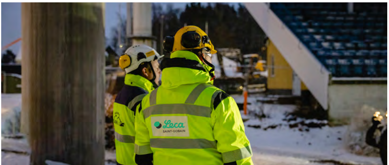
Maanrakennus Kivelä Oy's owner Ville Kivelä (left) and Leca Finland's Area Sales Manager Marko Jelonon discussing the progress of the project.
