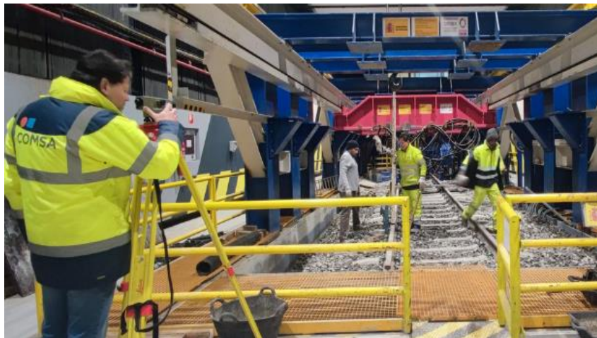
Figure 44.- Levelling of railway track sections.
