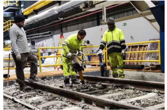
Figure 43.- Left: Ballast layer with sleepers, rails and fastening system. Right: Hand-held vibrator for ballast compaction
