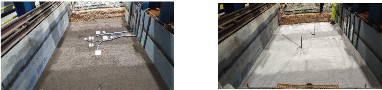
Figure 33.- Left: LECA embankment top with instrumentation. Right: Geotextile over LECA embankment
