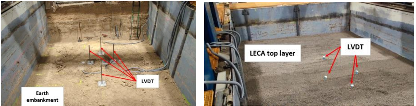
Figure 94.-Installation of LVDTs to measure LECA embankment vertical displacements
