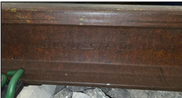
Figure 17: UIC 60 rail used in railway track section
