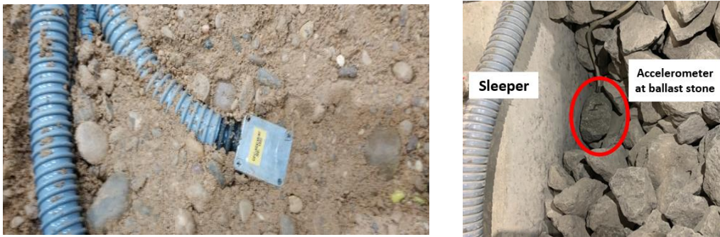
Figure 49.- Example of an accelerometer installed inside the railway track section (left) and instrumented ballast particle (right)
