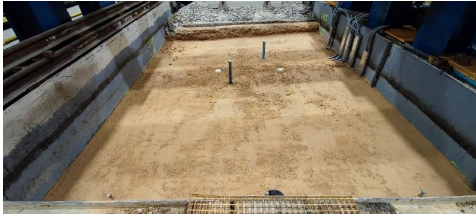
Figure 36.- Top of the form layer after construction
