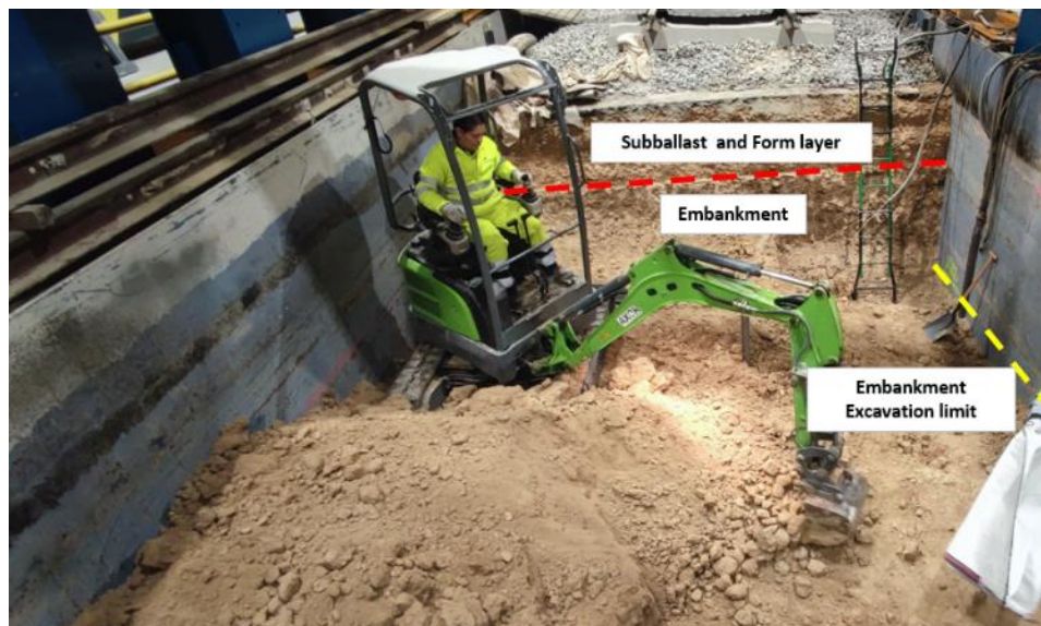
Figure 22.- Excavation of the embankment using machinery
